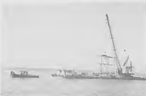
ONE OF two structures that support No. 3 Finger Pier's free-standing loading arm is transported by a Raymond barge from the assembly area near the Gasoline Docks to the pier's breasting island.
